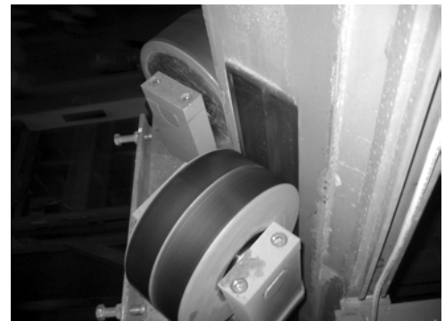
Floor-to-floor elevator guide wheel of NYTEC-HS
